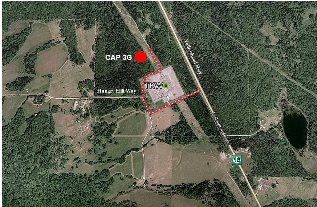
Figure 3: Capacitor Site 3G Location and Access
