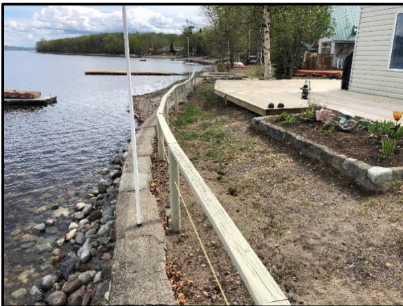
Retaining wall/ Natural Boundary
