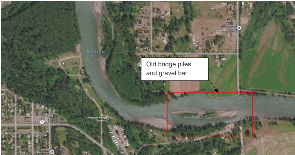
Figure 28: Current Photo at the Old Bridge Location (Bing Maps)
