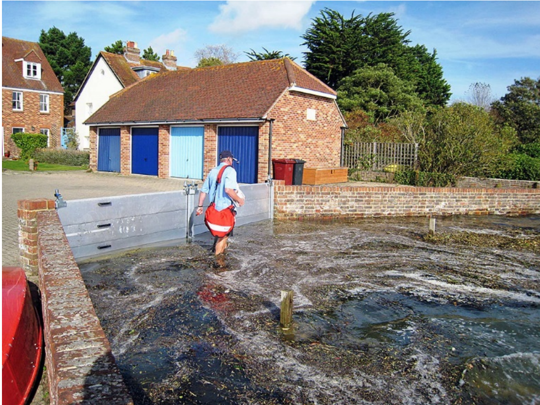
Figure 19: Example Flood Barrier (Constructed in a Wall)
