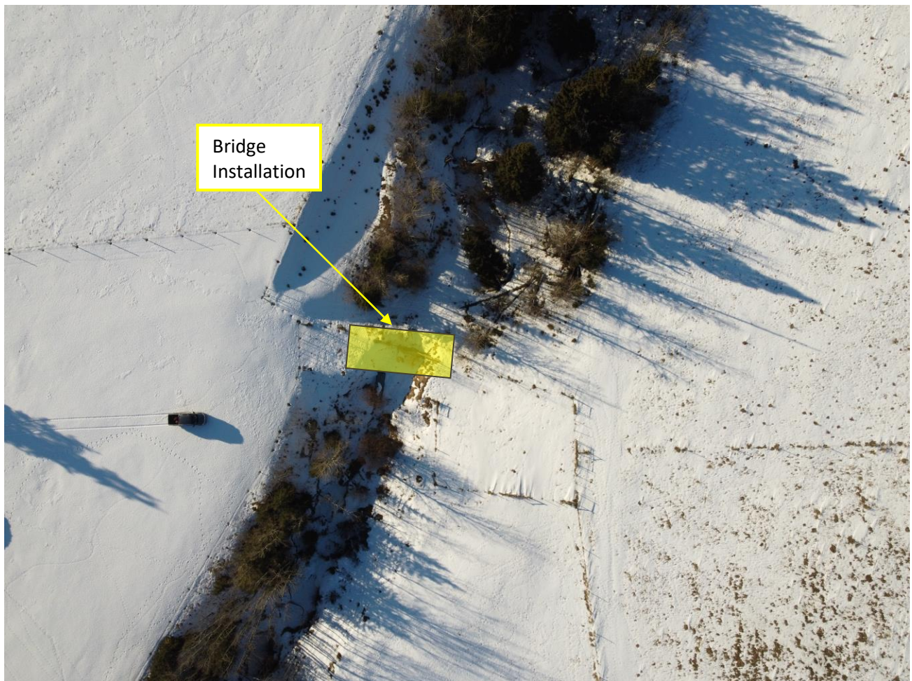
Figure 3. Site 2. Bridge Installation.
