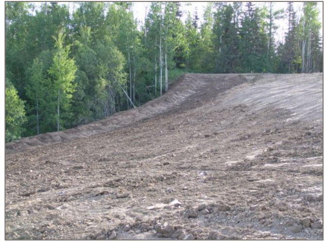
Photo 2-2: Closure of Historical Fort St. James Landfill (photo by RDBN 2010)
