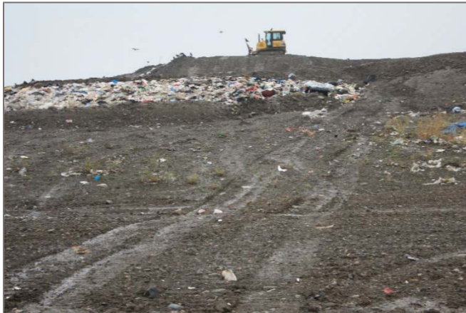
Photo 2-10: Clearview Landfill Active Face (photo by Tetra Tech 2017)
