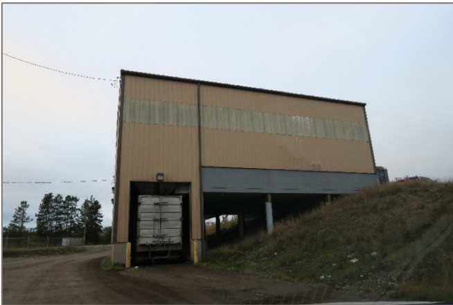
Photo 2-6: Smithers Transfer Station Trailer (photo by Tetra Tech 2017)
