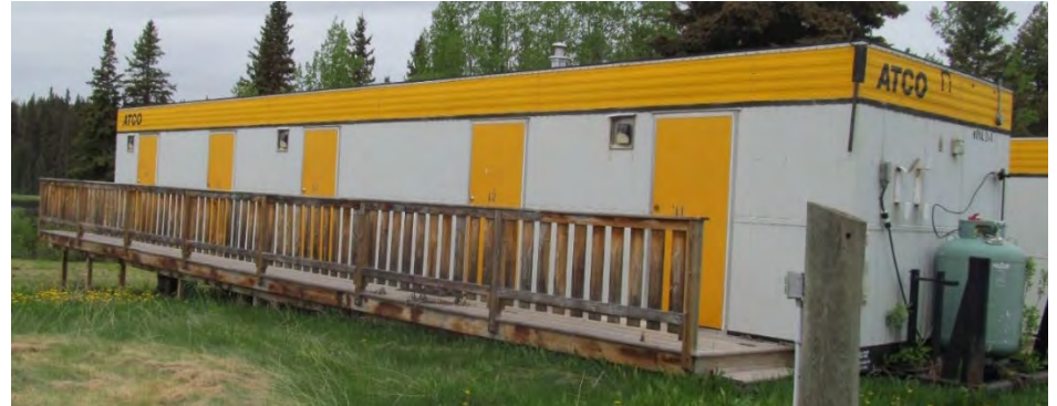
Photo 8: Staff housing in ATCO trailers, front view [17 cont'd]
