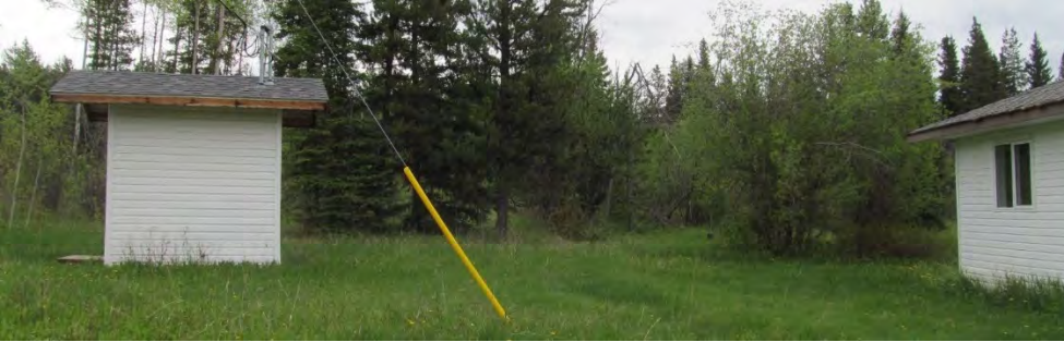
Photo 13: Power distribution shed, near boys bunkhouse [4]
