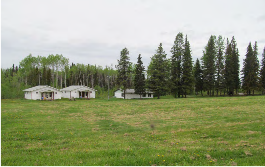
Photo 17 & 18: Girls bunkhouses and laundry room/staff room & caretaker house/ kitchen/dining hall building as viewed from centre of camp
