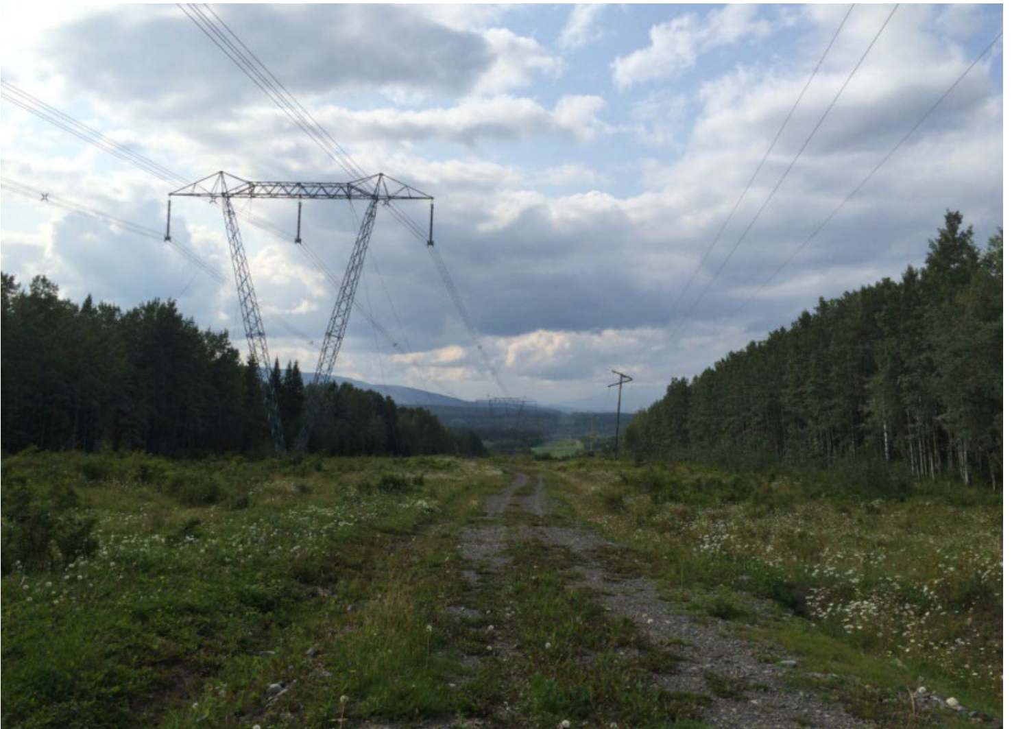
Figure 3 - Right of Way corridor looking northwest
