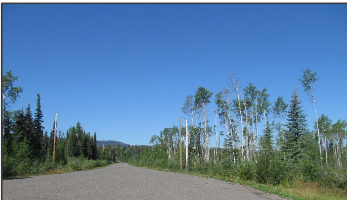
View of Clearview Drive from Dead End
