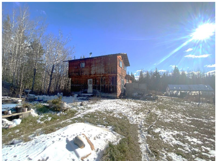
Photo #12: house (front view from driveway)
