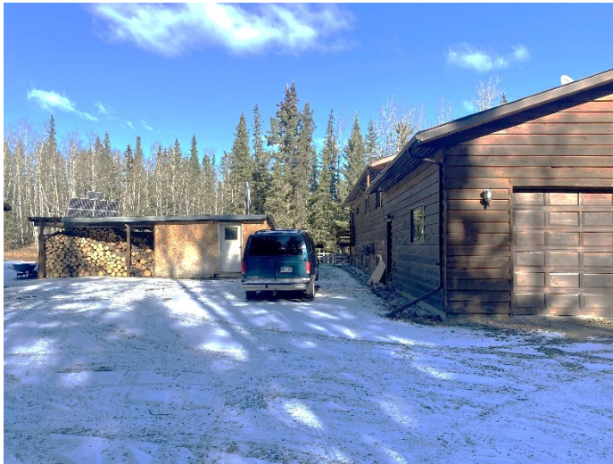
Photo #9: storage shed/wood storage
