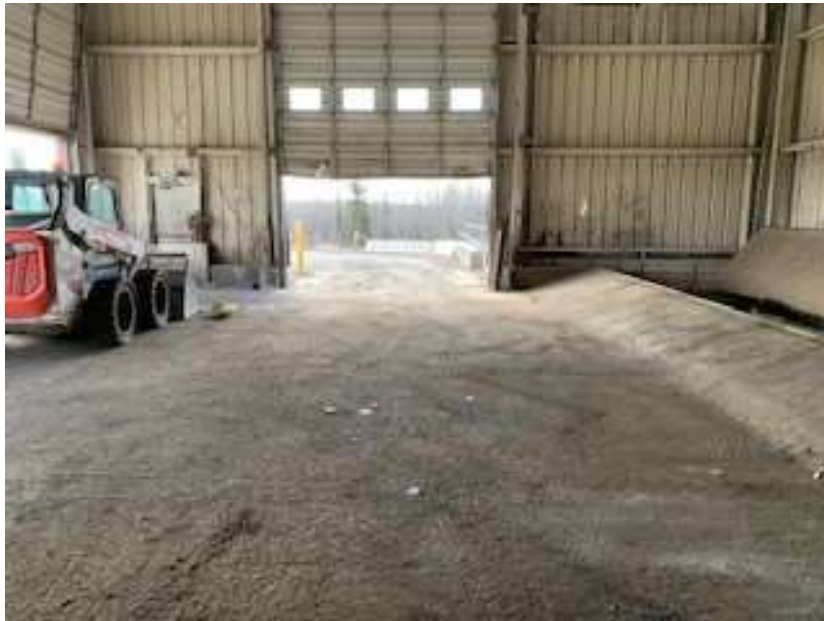
Figure 3 - Tip floor facing south
