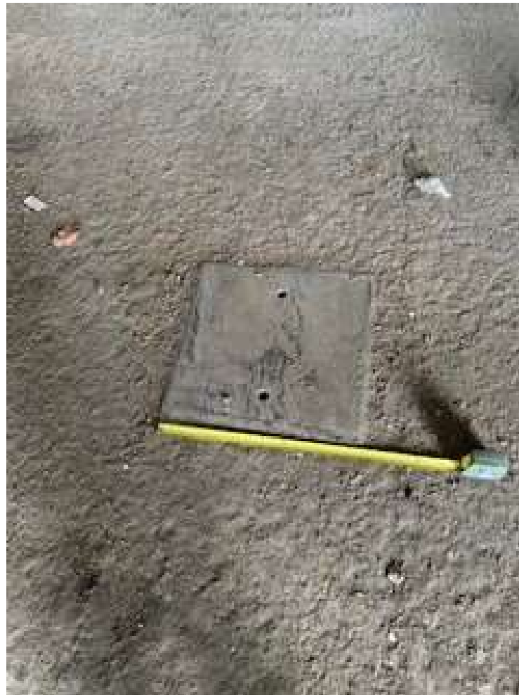
Figure 6 - 20" x 20" Floor drain covers plate (can be replaced or re-used)
