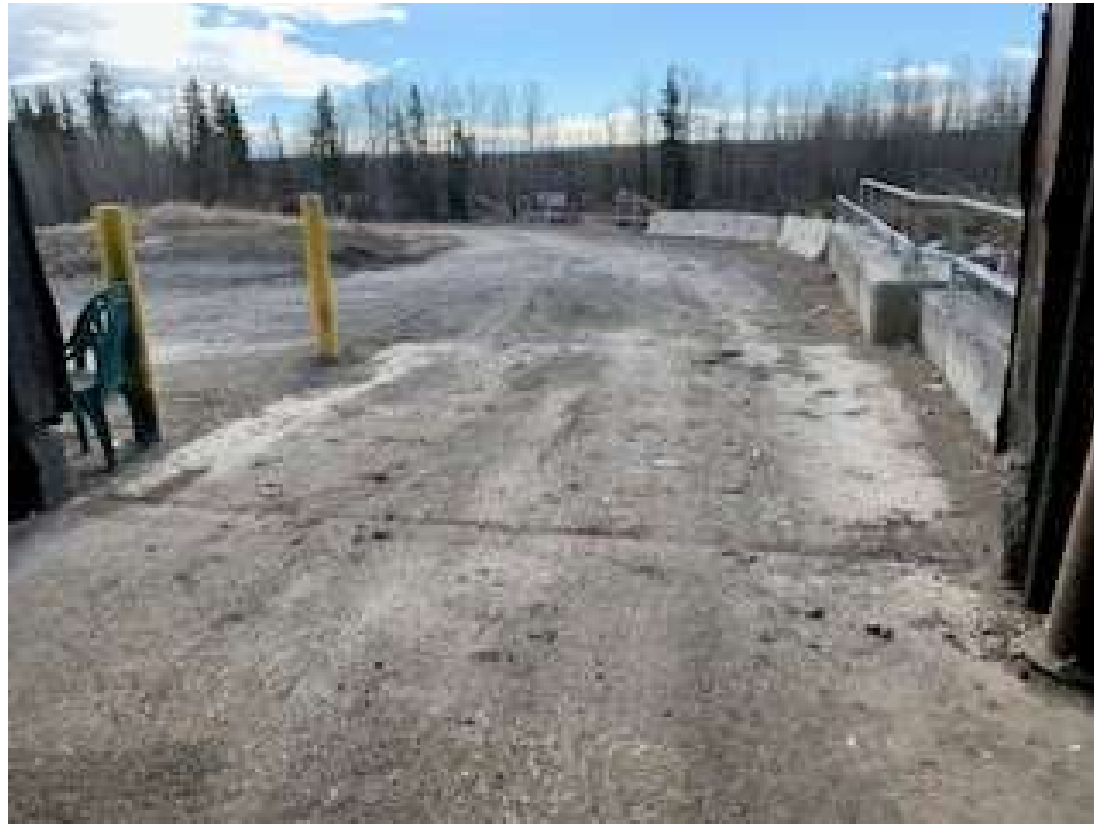
Figure 2 - Apron Facing South
